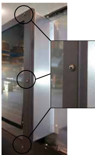
Figure 16. Step 3 (Removal of Door Frame)
